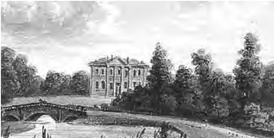
Atherton Hall and Lions Bridge c. 1726.
