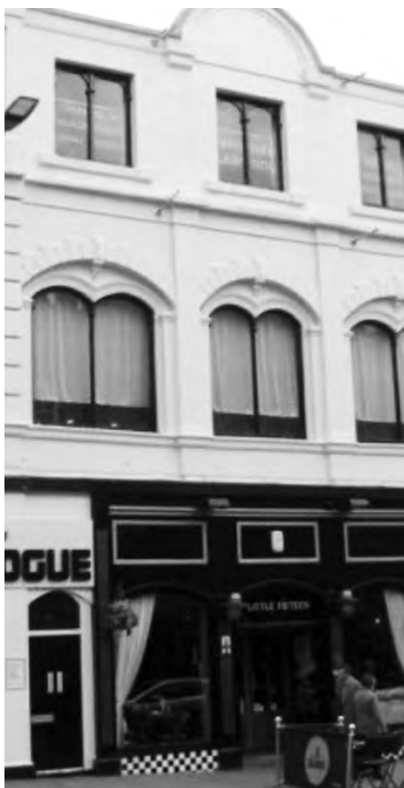
Meek's Building, 17-19 Wallgate
