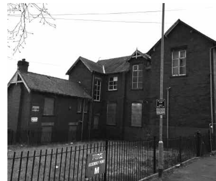
Tyldesley Primary School prior to demolition
