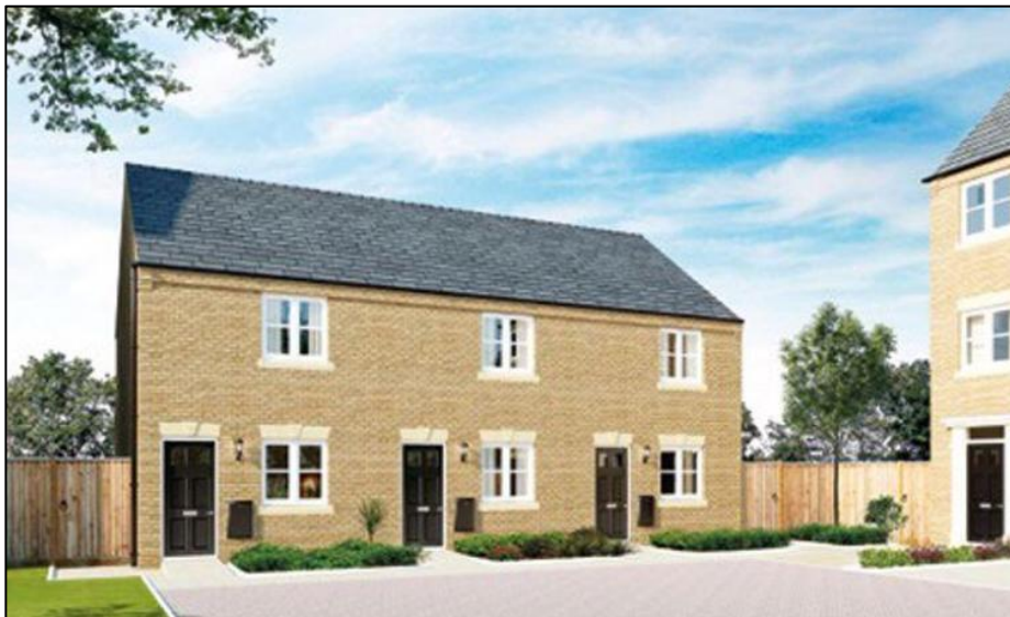
Figure 6.8 – Lathom Grange terraced house
