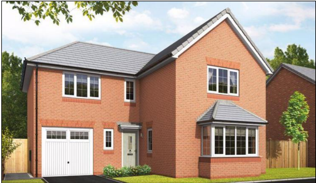
Figure 6.16 – Property photos at Rectory Woods
